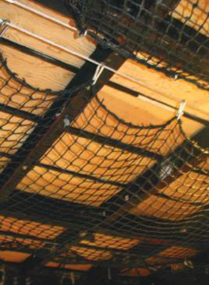
The Santa Fe Opera's trap room safety netting. Photo by Paul Horpedahl.
